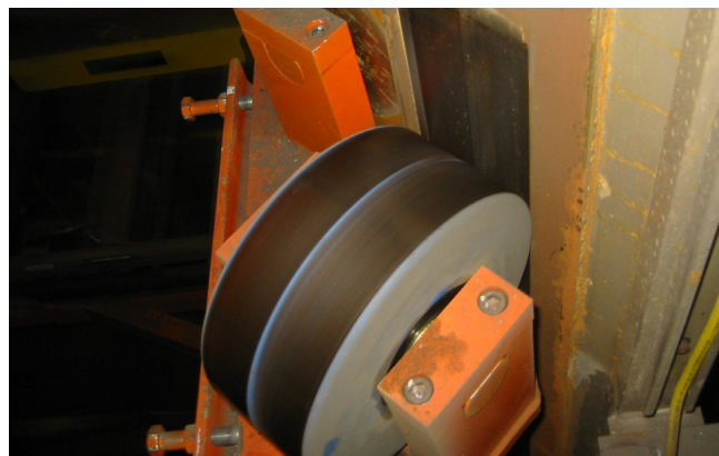
Floor-to-floor elevator guide wheel of NYTEC-HS
